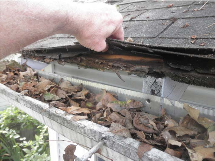
13 wood under shingles rotted, next photo too
