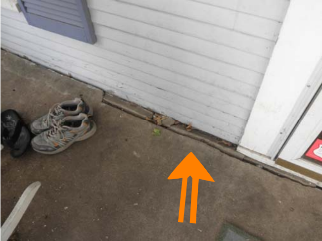
cracked + flashing missing
