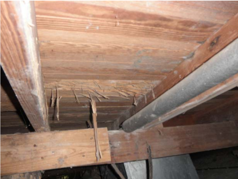
21 old termite dmg. to floor under DR
