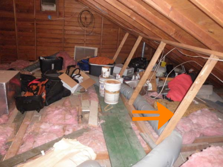
17 lots of stuff in attic, some may be from previous tenants note: rafter supports don't comply with current stds. but ARE adequately supporting the roof
