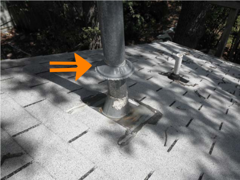
11 lower flashing 6"
