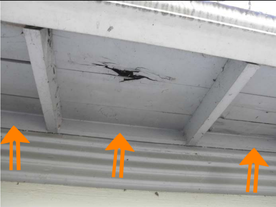
14 note missing air vents as well, arrows
