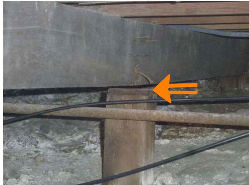
5 pier not supporting beam
