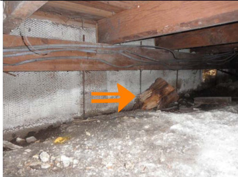
4 pier has fallen over leaving beam unsupported
