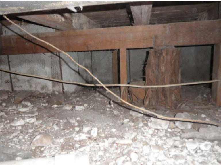
2 earth to wood contact WILL attract termites. note wires hanging down loose and original cedar piers in use
