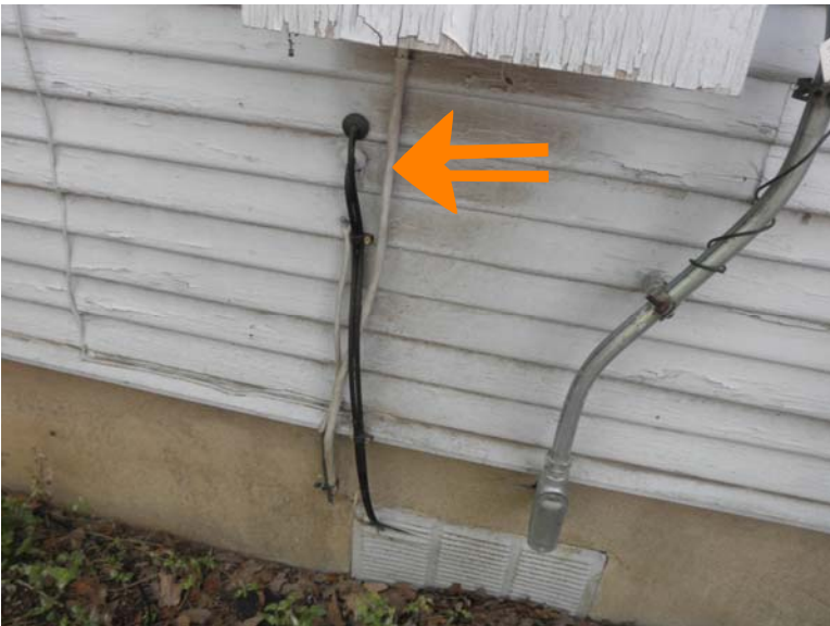
27 wiring under breaker panel not in conduit
