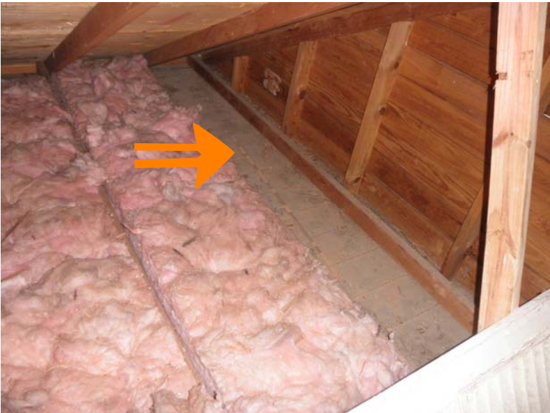
15 insulation missing over back BR
