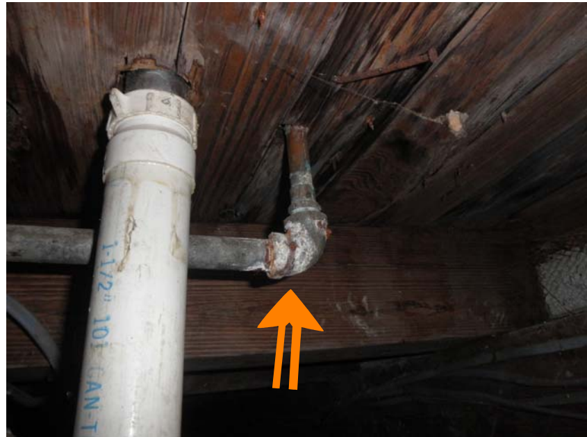
31 more corroded pipes, this is under bath
