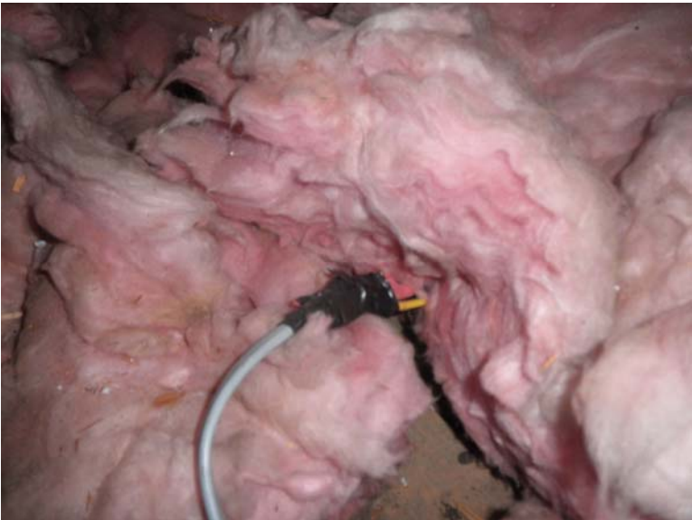
24 wire splice not in junction box over front BR
