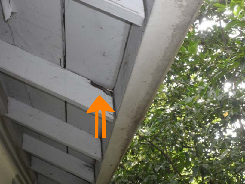
19 minor rot to front rafter "tails"
