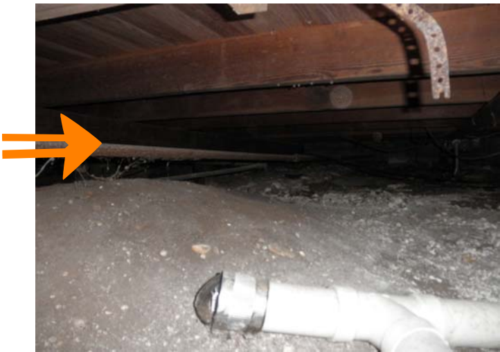
22 loose gas line under home, needs to be strapped up
