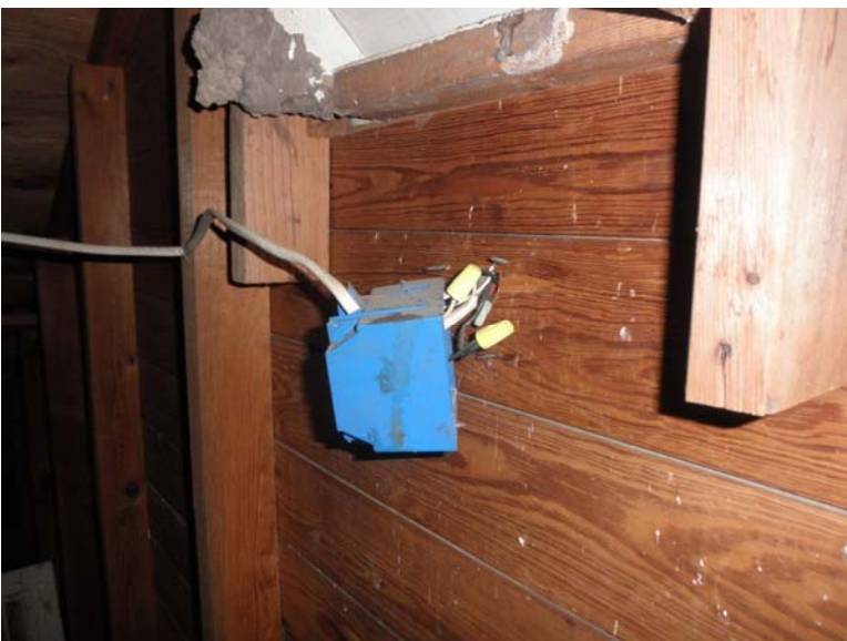
26 open wiring box at right side of attic
