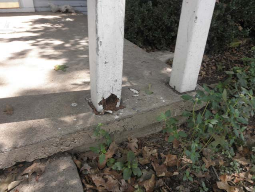
18 wood rot to front porch posts + brackets under them are missing
