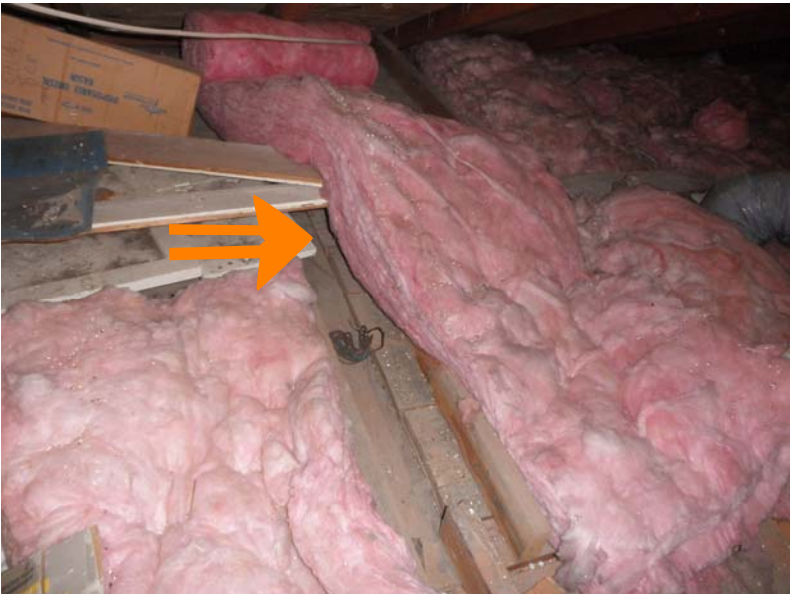
16 loose insulation, must lay FLAT on the ceiling to have any effect
