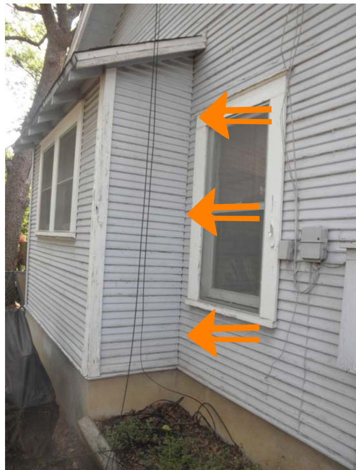
20 caulk siding gap on left
