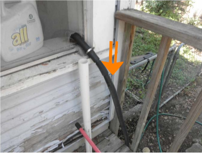
34 washer drains to yard
