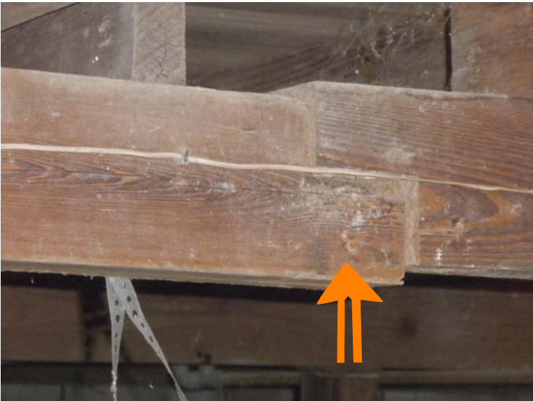
1 need pier under beam splice under DR
