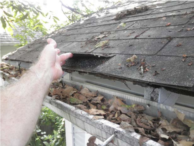
8 edge shingles not glued down, note full gutters
