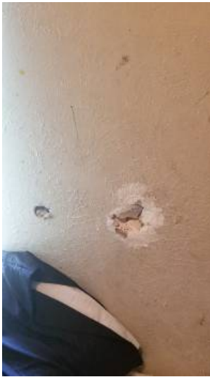
damaged sheetrock left front bedroom
