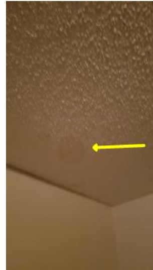
water stain on ceiling sheetrock.
