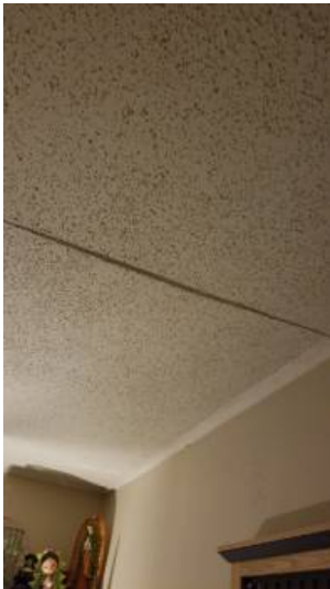
converted garage ceiling sheetrock sagging.
