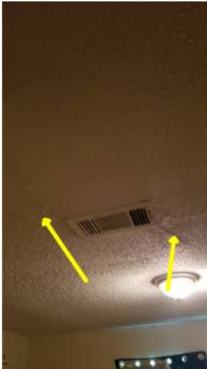
ceiling sheetrock cracked and sagging
