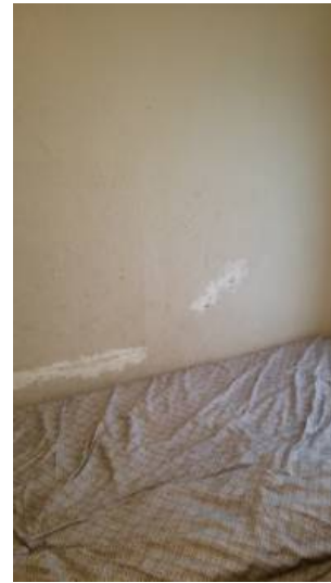
damaged sheetrock left front bedroom.
